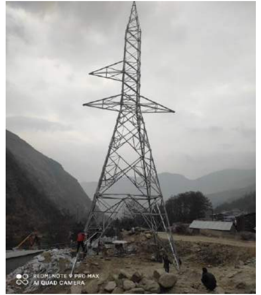
Erected Transmission Line Tower
