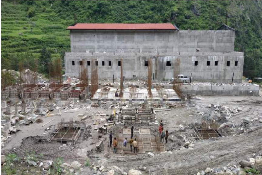
Switchyard and Powerhouse Area
