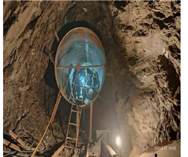
Penstock Installation Work
