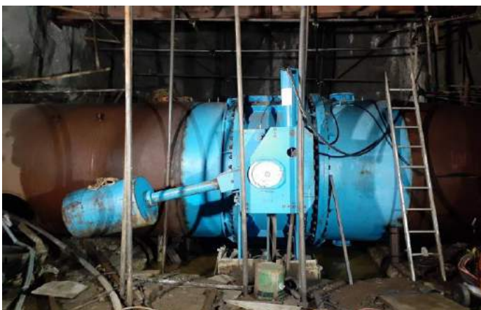
Penstock Valve Installation
